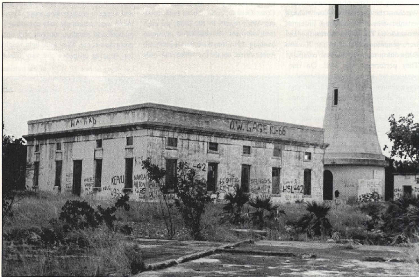
Many years ago this served as the quarters for the lighthouse keepers; it now provides 5 stations for our DXpeditioners.
